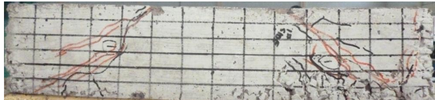
Figure 6: Crack patterns of specimens
